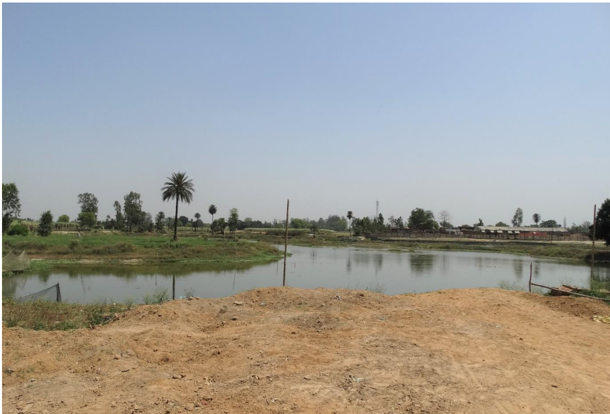
Image 18 : Earth Filling at Pond In Nangal [Looking Southeast]
