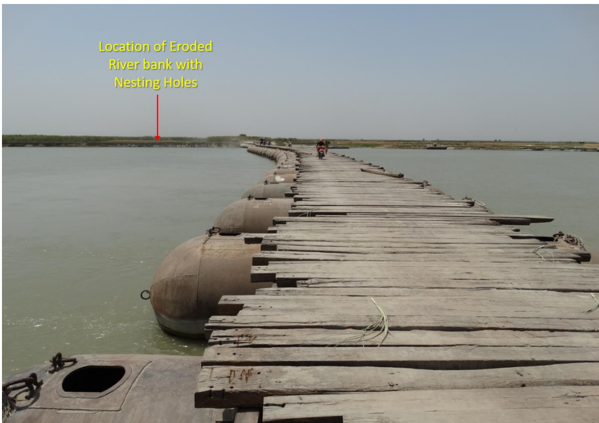
Image 57 : Temporary Pontoon Bridge Connecting Eroded River Bank
